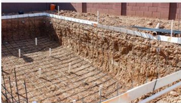
Structural Steel is the steel reinforcement that creates the backbone of your pool to give it added strength per the plans. It consists of a series of bars specifically engineered for your pool design requirements. At Lee-Sure Pool we use a steel in the top of the shell that is twice as thick as the industry standard. Because we believe that this type of investment should last a lifetime.
